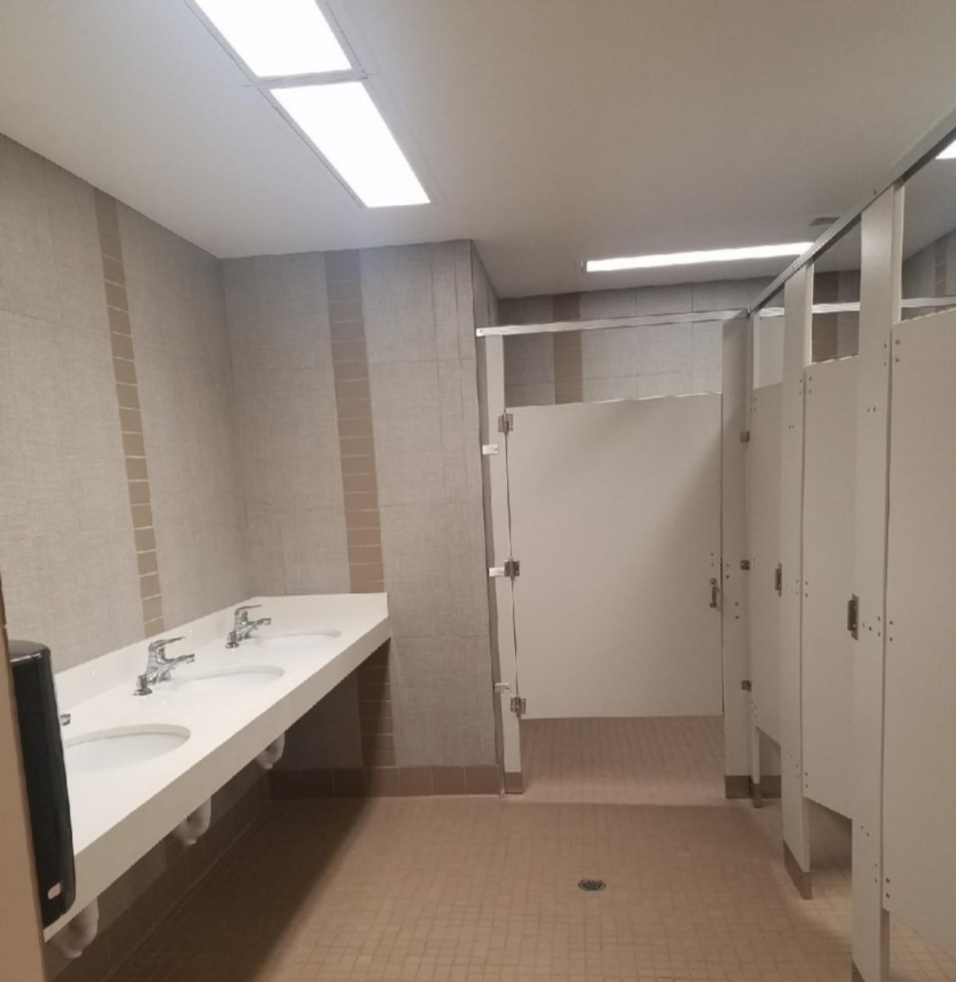
Bldg. 66 women's rest room renovation
