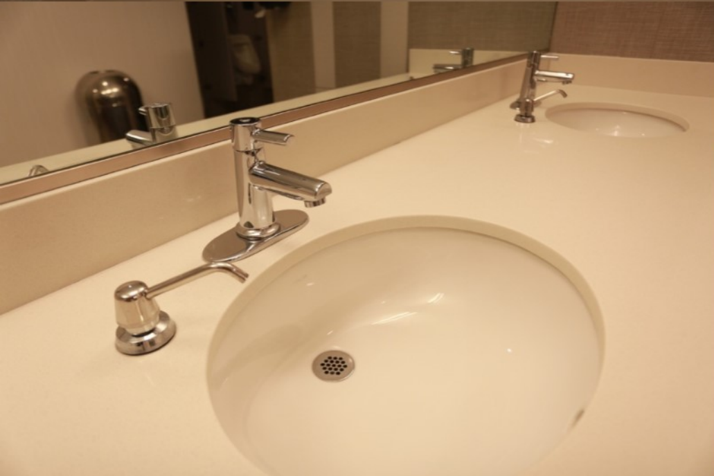
KW men's rest room renovation
