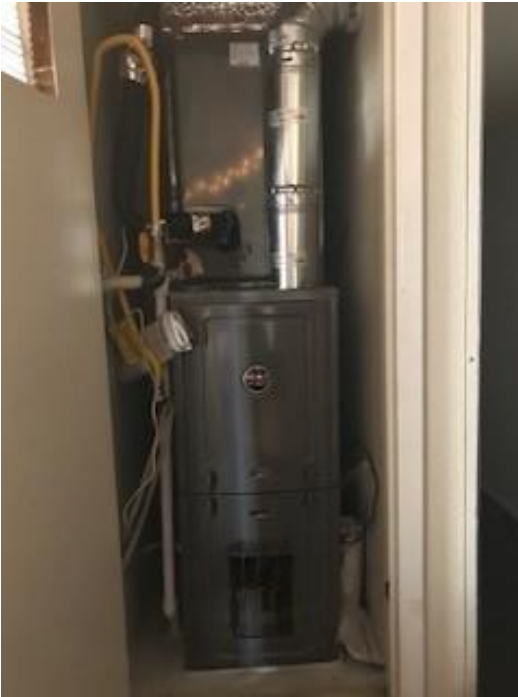
New Phase II HVAC
